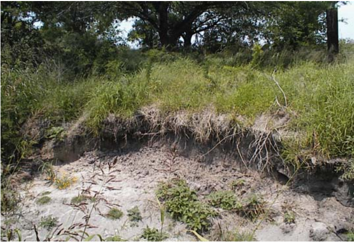
Prior to establishment of the riparian buffer, stream banks were subject to erosion by high velocity flows.
