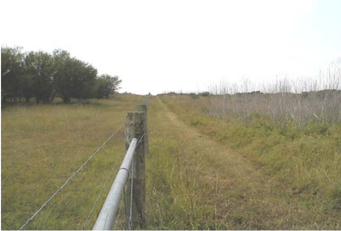
A barbed wire fence was constructed to exclude livestock from the riparian area (on right).
